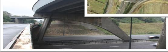
**The solution:** APA Concrete Repairs Ltd were involved in refurbishing the supporting structures as part of a central barrier replacement scheme on the M1 section. An extensive programme of concrete repairs was completed during limited night and weekend lane closures. These works included breakout by hydro-demolition, rebar replacement, installation of galvanic
